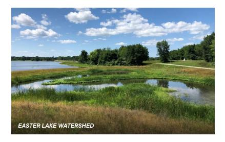
successful stormwater wetland provides continual treatment of pollutants through a slow settling process over time. While sedimentation of the wetland is inevitable in the long-term, there are proven methods for slowing down the rate of sediment entering and filling the waterbody. A pretreatment forebay should be considered, which is designed capture the heaviest sediment load as water enters the system. If dredging is
